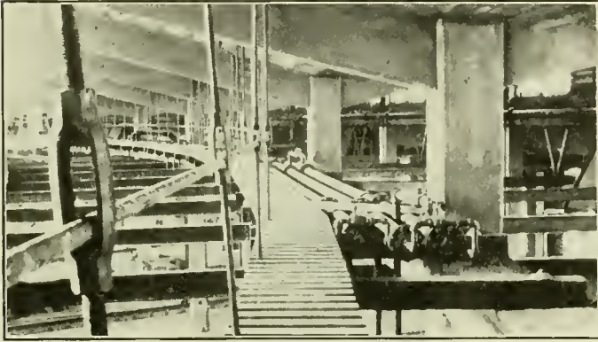
Inspection Runway in Gallery of Boiler Washing Plant
